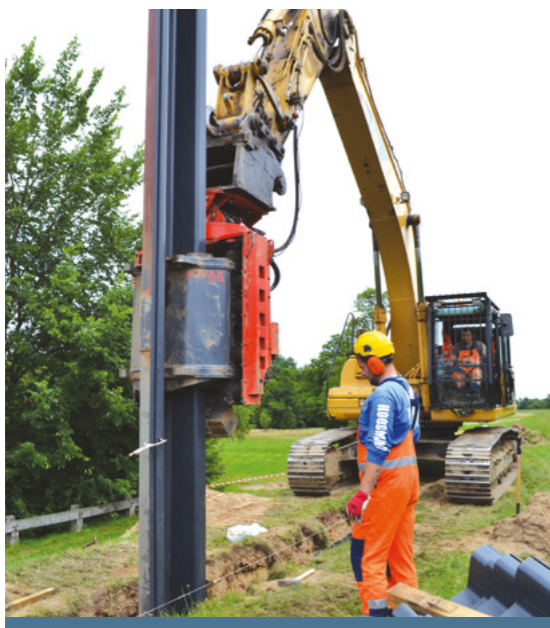
Hammering of a vinyl sheet pile using a steel mandrel
