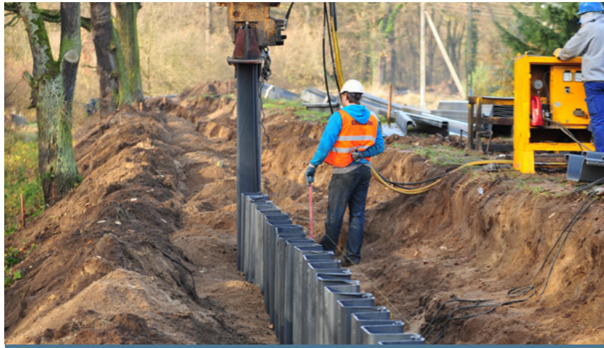
📍 Jelcz-Laskowice, Poland 📄 Modernization of embankments 🏗️ CW-610/9.0 📅 2013
