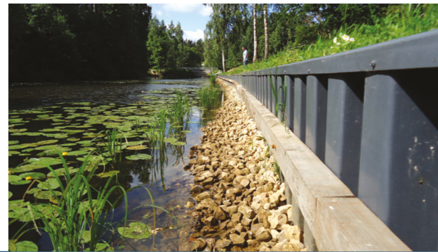
📍 Ryga, Latvia 📄 Reinforcement of river embankments and modernization of the flood-protection system 🏗️ CW-610/9.0 📅 2015
