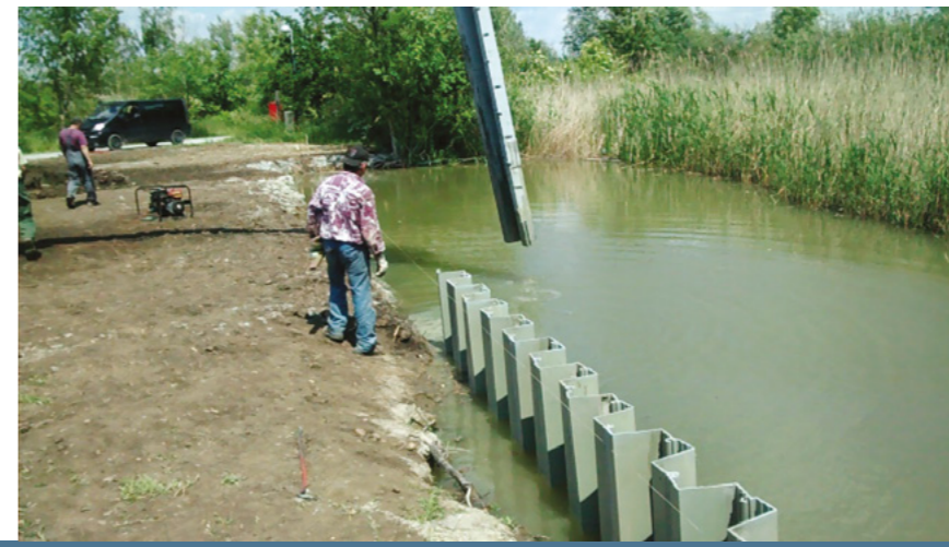
📍 Neusiedl am See, Austria 📄 Protection of the canal bank 🛠️ CW-580/9.0 📅 2014
