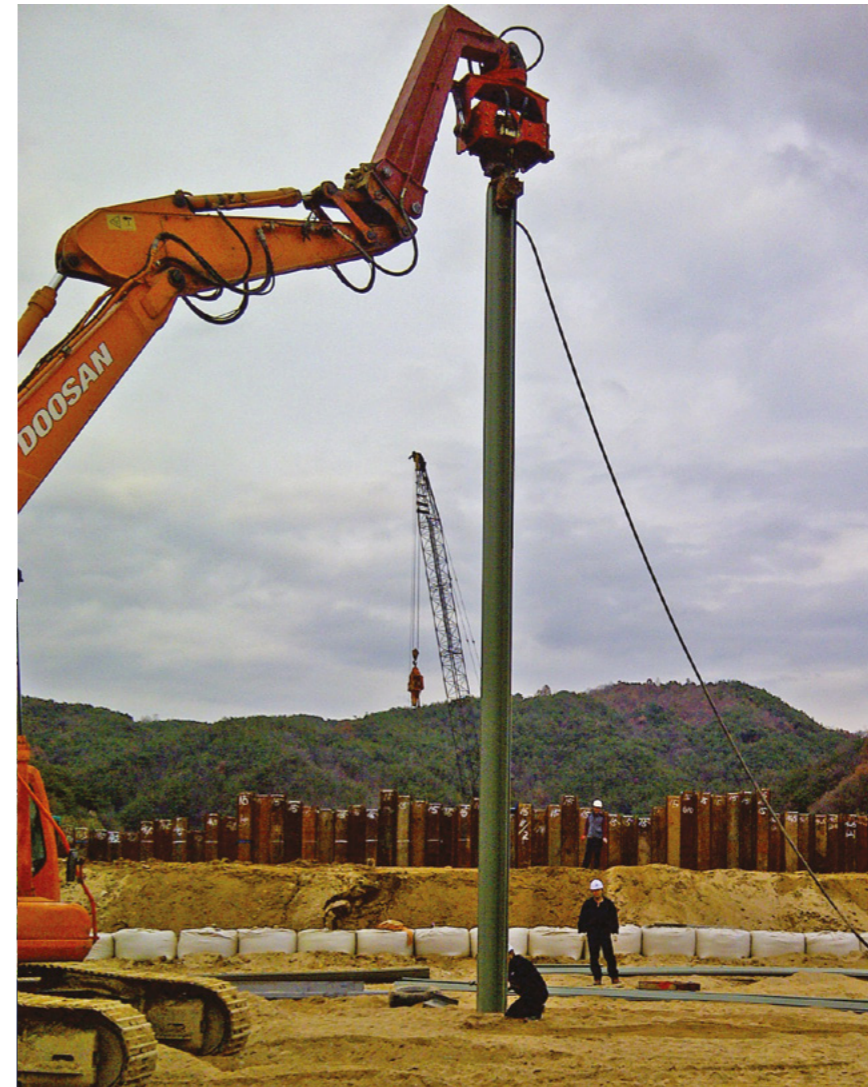
📍 South Korea 📄 Reinforcement of flood-walls 🛠️ CW-580/7.0 📅 2011
