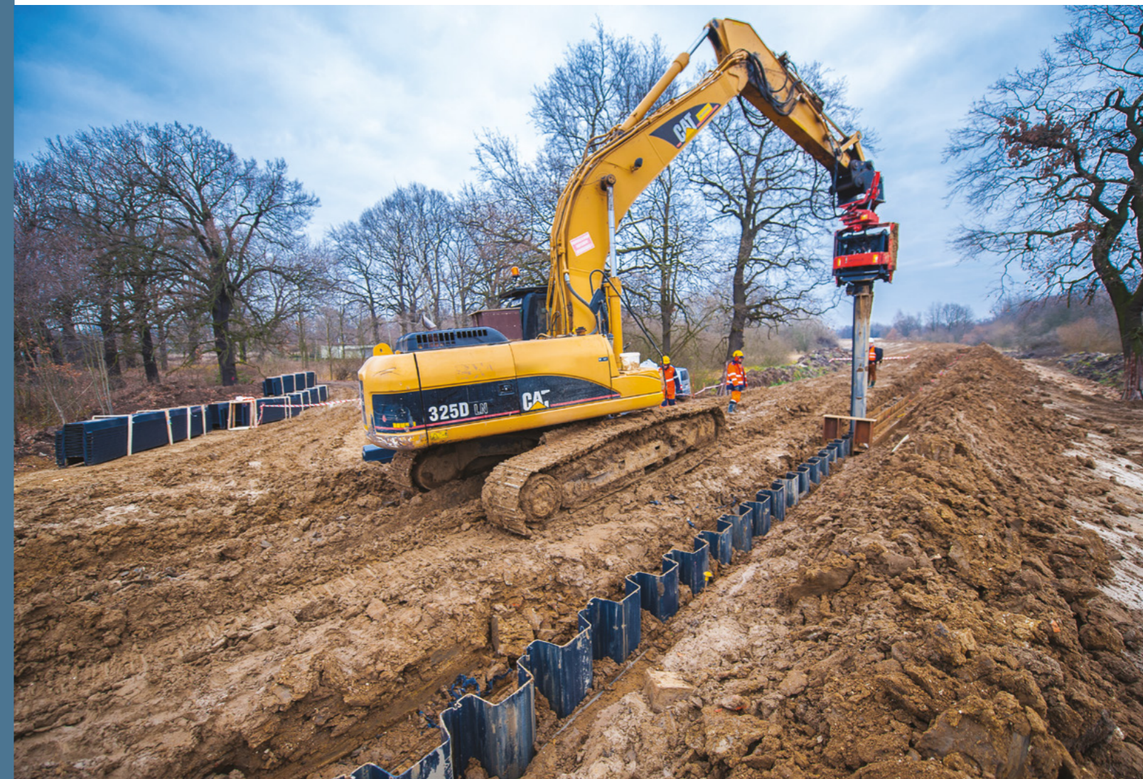
Vinyl sheet piling used to reinforce flood-walls.
