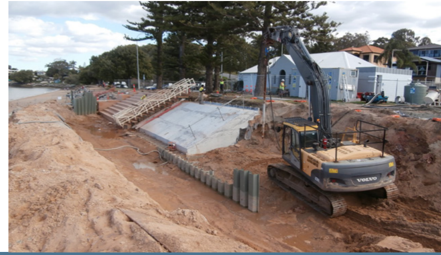
📍 Scott's Point, Australia 📄 Protection of the seawall 🏗️ CW-610/9.0 📅 2013
