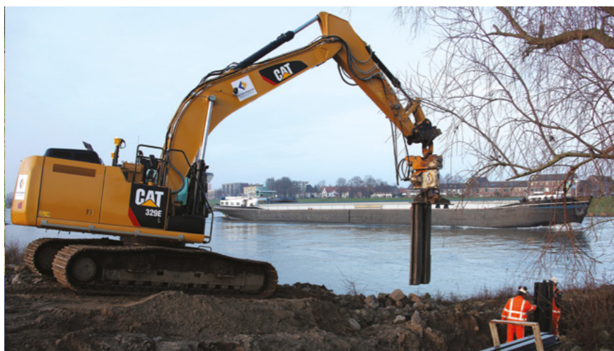
📍 Terwolde, Holland 📄 Protection of the canal bank 🛠️ CW-460/5.5 📅 2014
